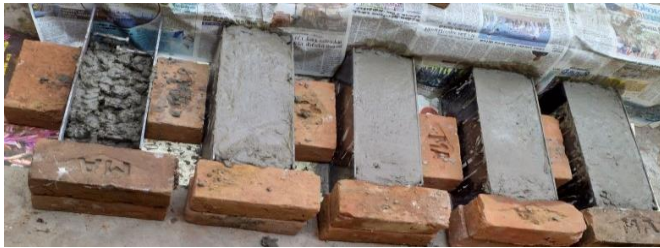
Figure 5: Casting of Beam
