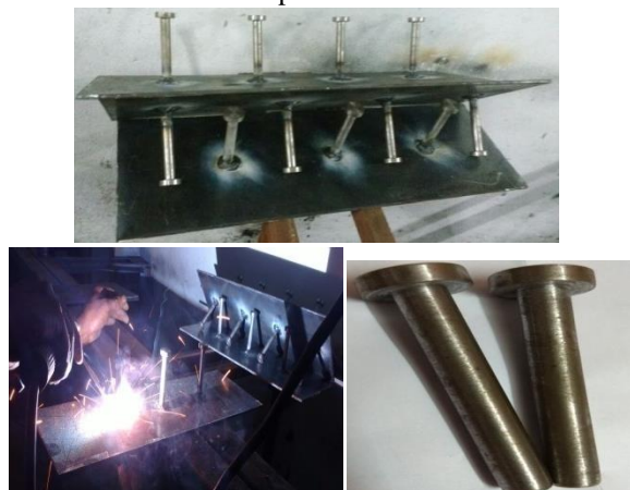
Figure 4: Welding of shear connectors in steel plate
